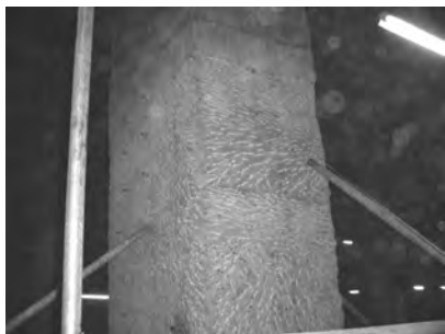
(a) Chipping of existing column face
