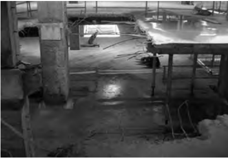
(a) Demolition of side core at B4 floor
