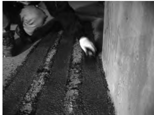
(b) Epoxy mortar casting
