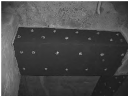
Fig. 7.21: Adding bonded steel plate in beams
