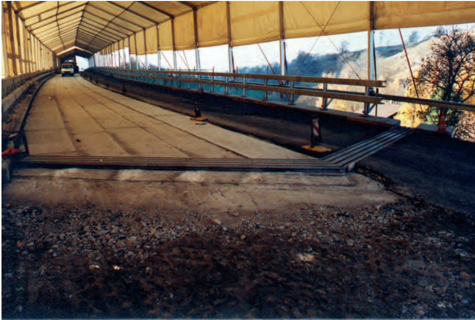
Fig. 2.10: Covered building site of the Chritzi Bridge repair
