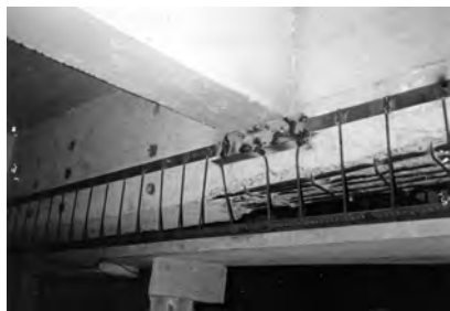
Fig. 5.15: Reinforcement detailing at beams
