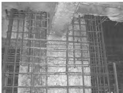
(c) Apply additional reinforcement
