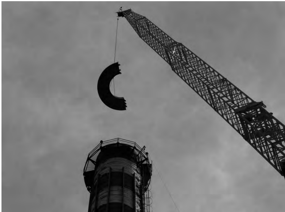
Fig. 6.12: Shaft top element installation
