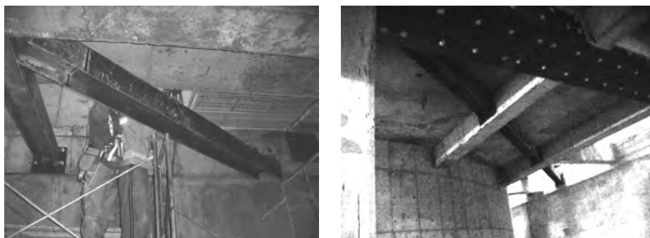
Fig. 7.14: Temporary shoring
