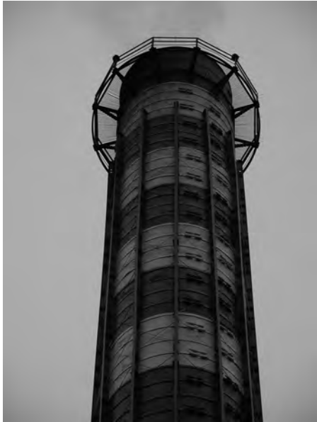
Fig. 6.5: The construction of steel strengthening of the upper part of the shaft
