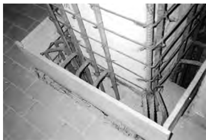
Fig. 5.16: Reinforcement detailing at column-foundation joint
