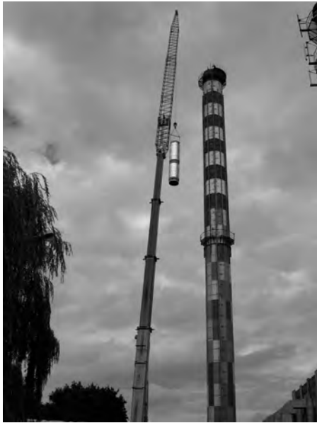
Fig. 6.11: Smoke conduit typical element installation
