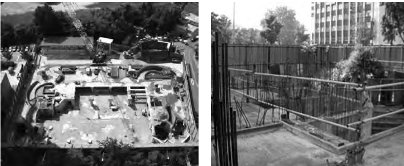
Fig. 7.9: Site view before rehabilitation
