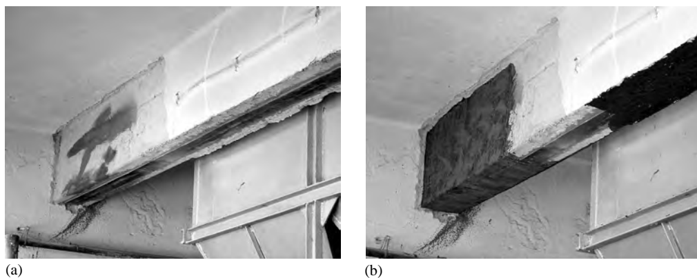
Fig. 5.20: CFRP application for beams: (a) longitudinal strips; (b) transversal sheets
