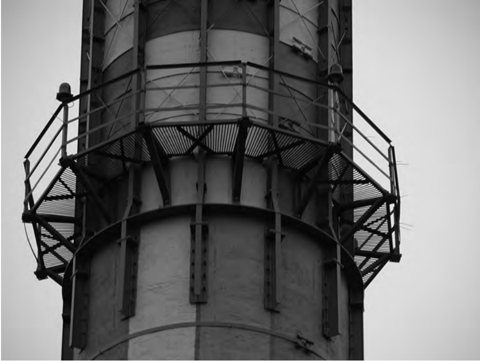
Fig. 6.6: The detail of resting the steel members on the additional RC jacket
