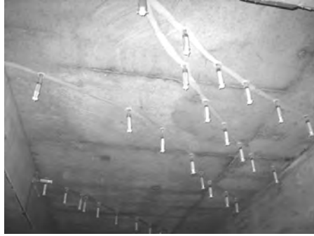
(b) Epoxy injection
