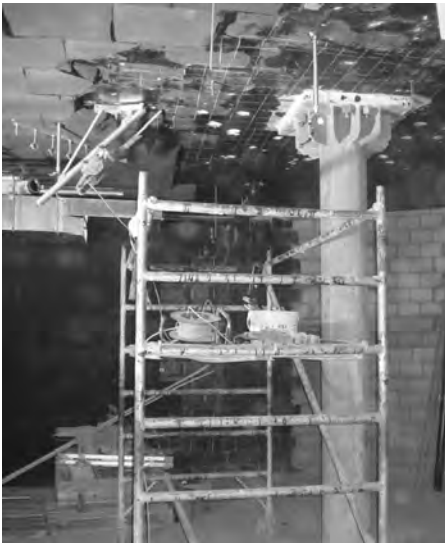
Fig. 4.21: Mobile scaffold and hammer drill anchored to the slab
