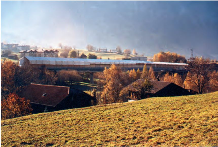
Fig. 2.2: Chritzi Bridge in its environment during the repair
