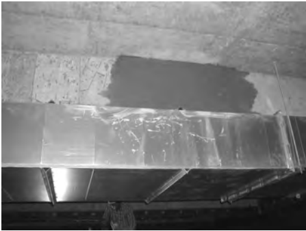
Fig. 7.12: Patching method at the honeycomb and concrete spalling region
