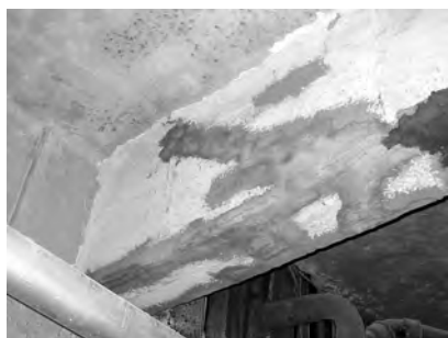
Fig. 5.17: Surface repair and preparation before CFRP application
