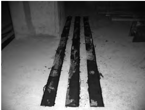
(a) Steel plate embedment above the beam
