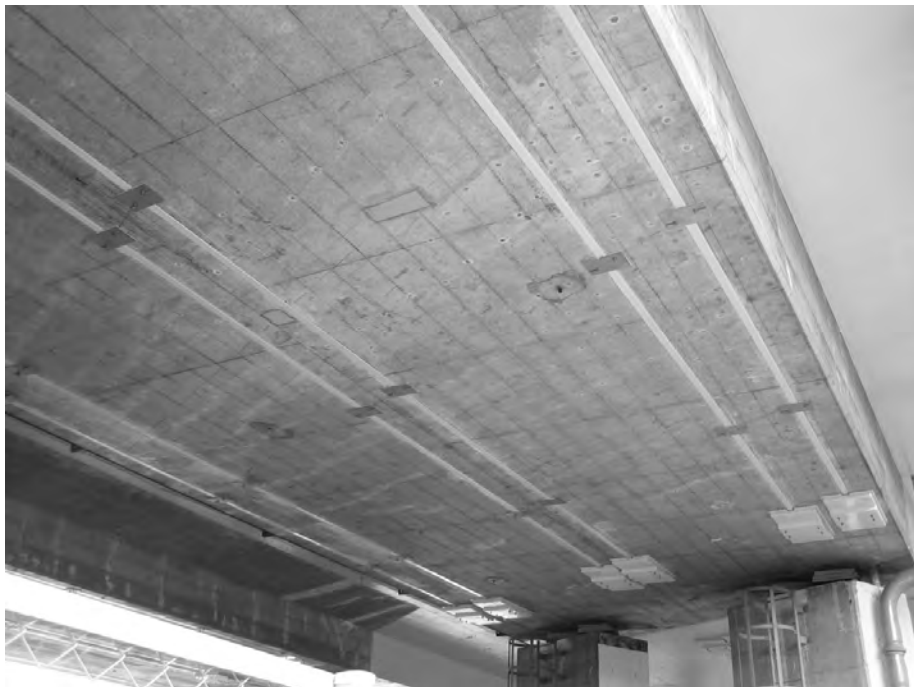
Fig. 3.8: Applied tensioned CFRP strip
