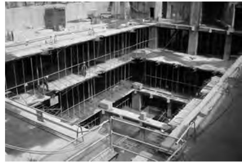
(b) Demolition view at 1 st floor
