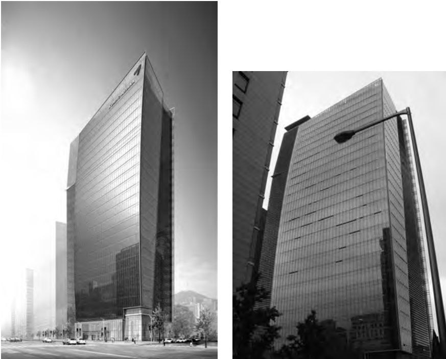
Fig. 7.2: Perspective and real view of the rehabilitation building
