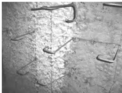
(b) Anchoring of dowel
