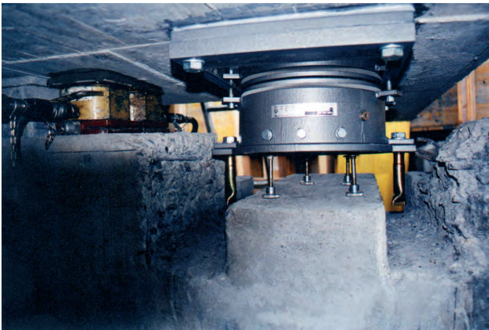
Fig. 2.7: Uplifting of the bridge during replacement of the abutment bearings [1]
