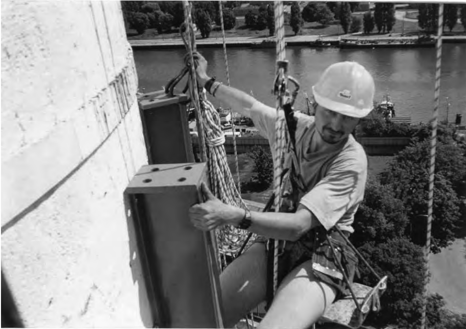
Fig. 6.9: Assembly of the elements of the shaft steel strengthening
