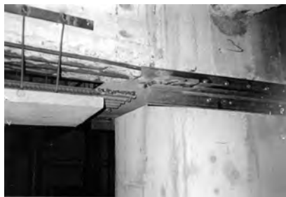
Fig. 5.14: Anchorage detailing at beams end
