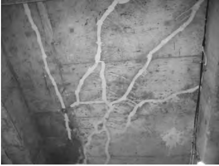
(a) Surface caulking before epoxy injection
