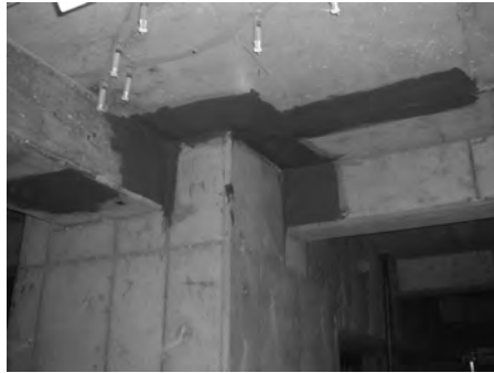
Fig. 7.12: Patching method at the honeycomb and concrete spalling region
